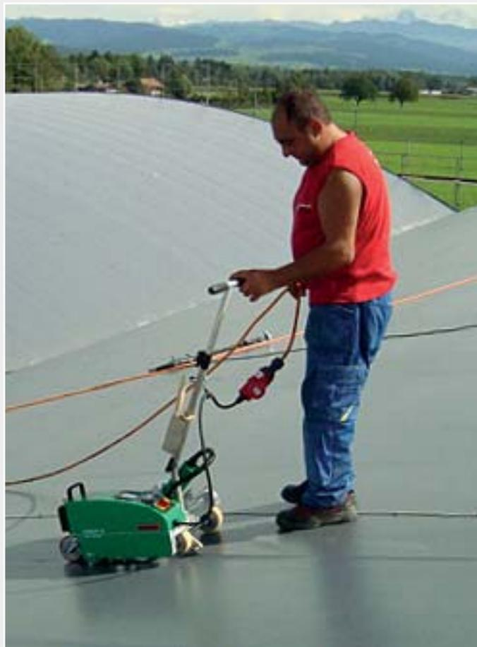
*The VARIMAT V2 – for faster welding of polymeric waterproofing membranes.*
