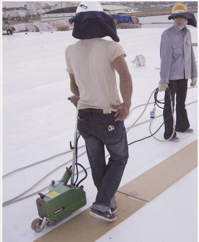
*UTo compensate for the pressure, welding was carried out walking on boards.*
