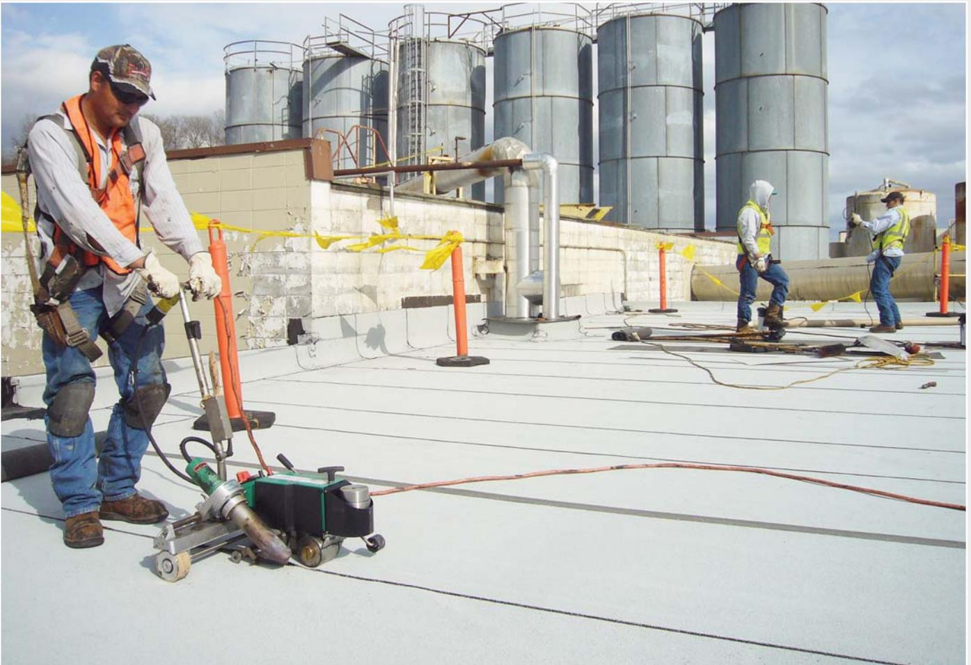
Safe and secure welding of bitumen sheeting with the BITUMAT B2.
