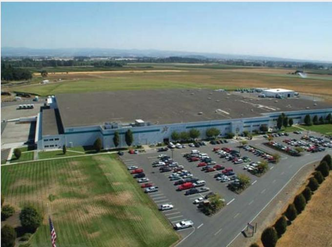
*The massive 420,000-square-foot ballasted roof atop Food Services of America's Woodburn, Ore., distribution center had seam failures tearing as fast as 50 feet per week.*
