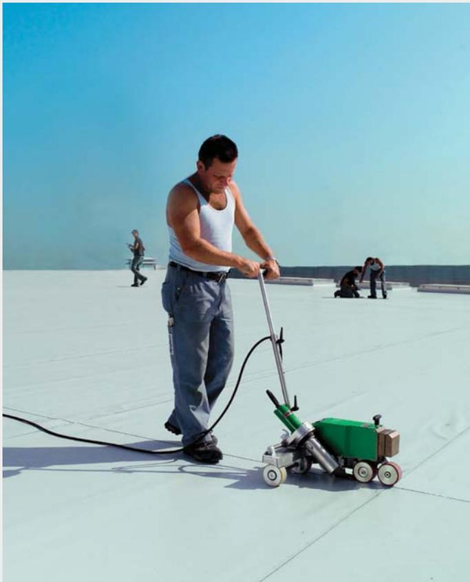
**With the VARIMAT V walk welder, Columbia River Roofing was able to weld 22,000 to 25,000 square feet per day.**
