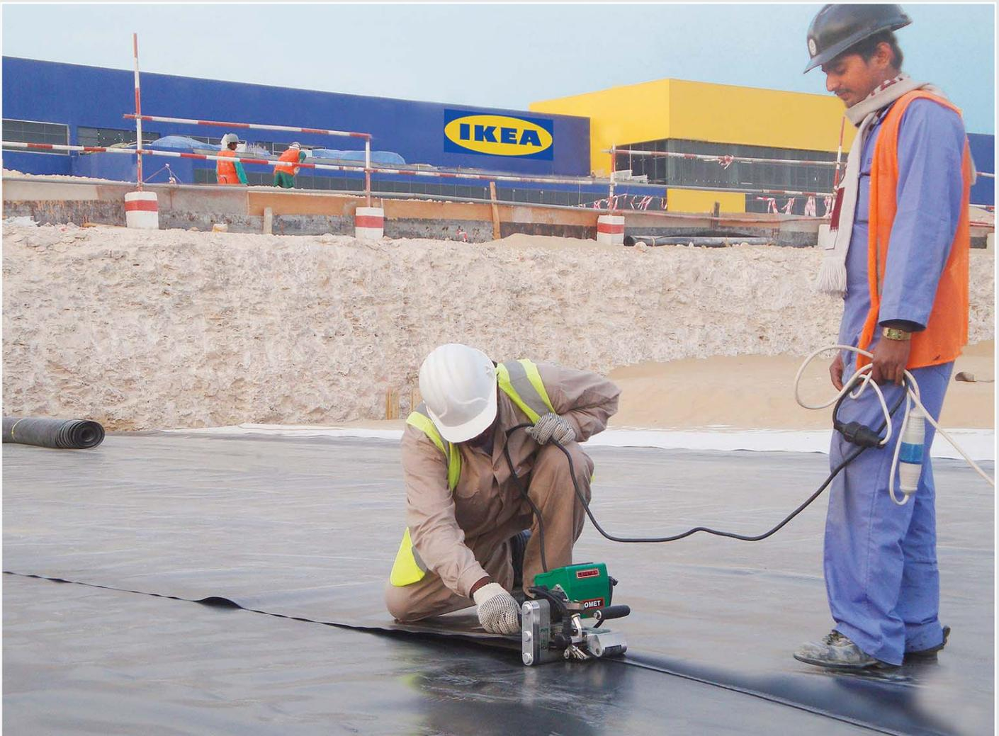
*Easy operation and clean working with the COMET hot wedge welder.*
