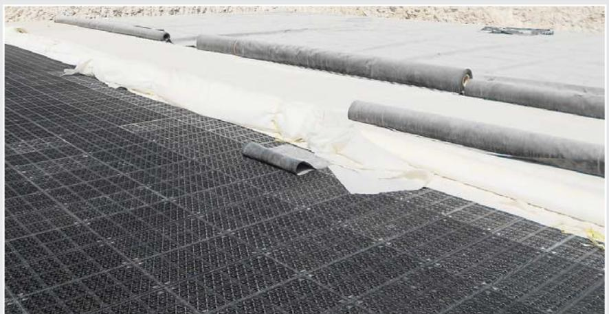
*Stacked polypropylene modular tanks in the foreground, behind the two-layer system structure with geotextile and HDPE sealing sheet.*
