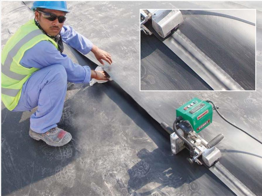
*The COMET welds two parallel weld seams with up to 1000 N.*
