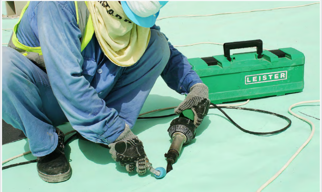
All details are welded with TRIAC AT hot air hand tools.
