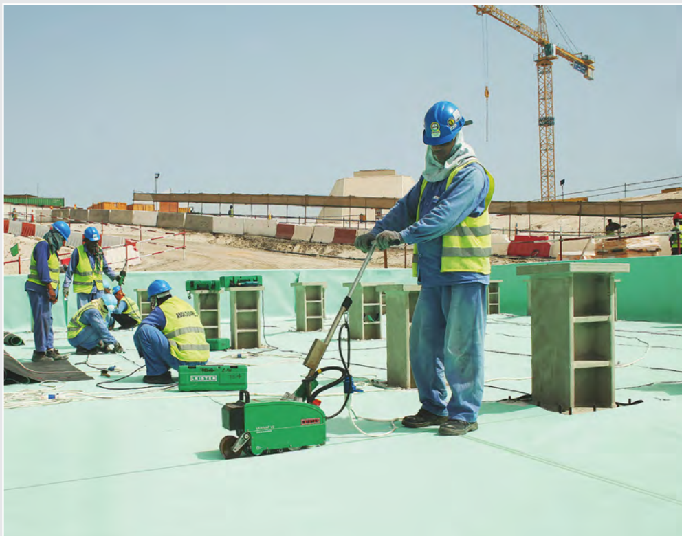
Welding of the upper layer with Leister's VARIMAT V2.
