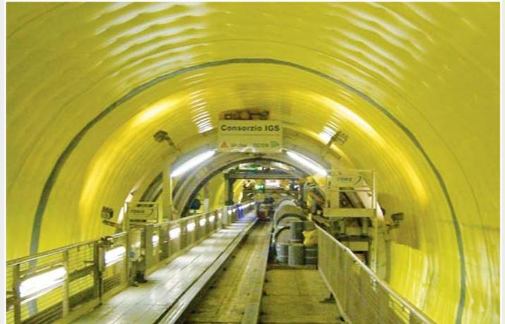
*Finished tunnel seal. The individual sheets are welded in parallel.*
