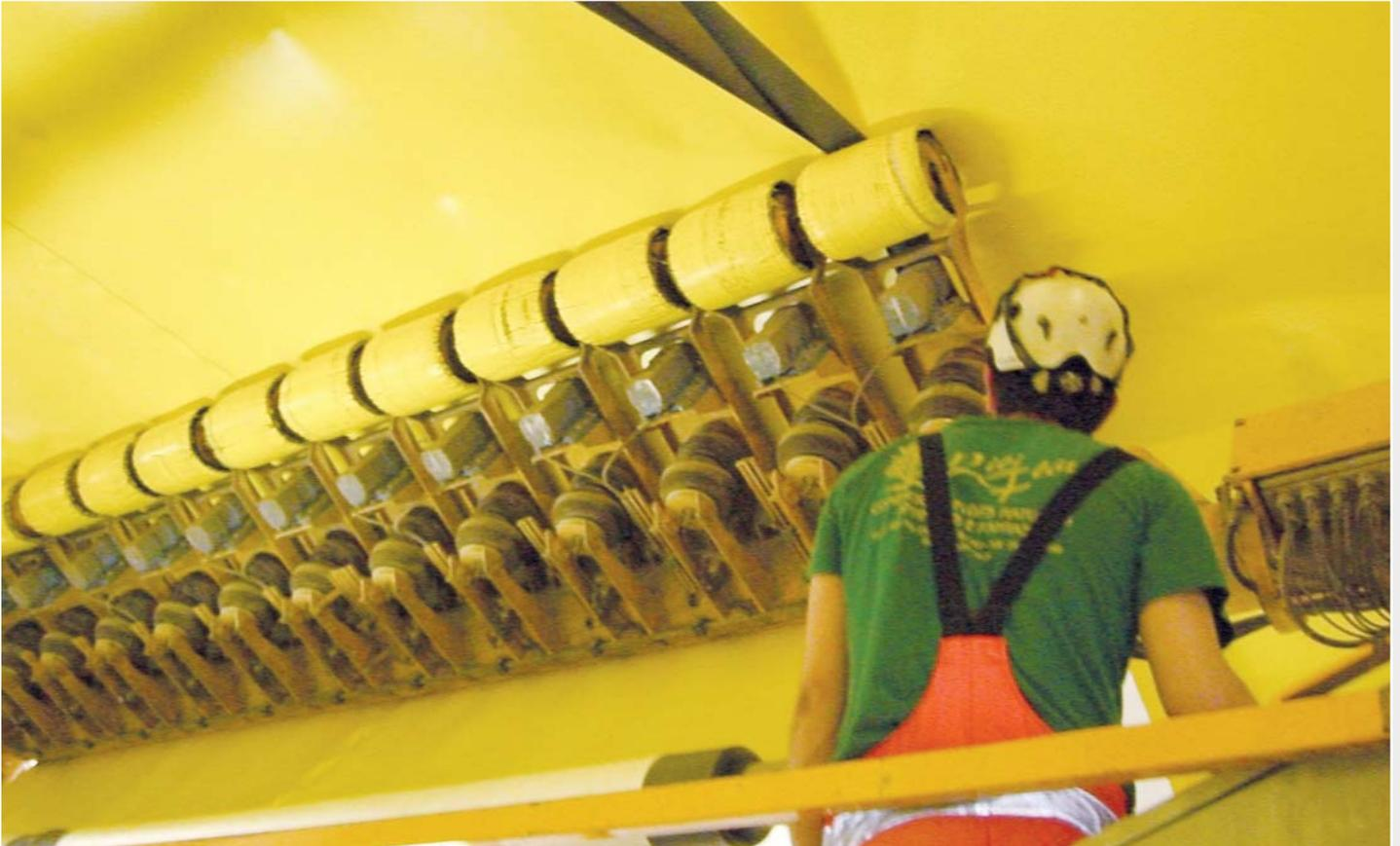
*Mechanical application of the prefabricated, 4.30 m wide plastic sealing sheets onto the Velcro-backed discs located below. Welding is then carried out.*
