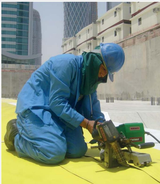
*TWINNY T welding machine welding a double weld seam with test channel.*
