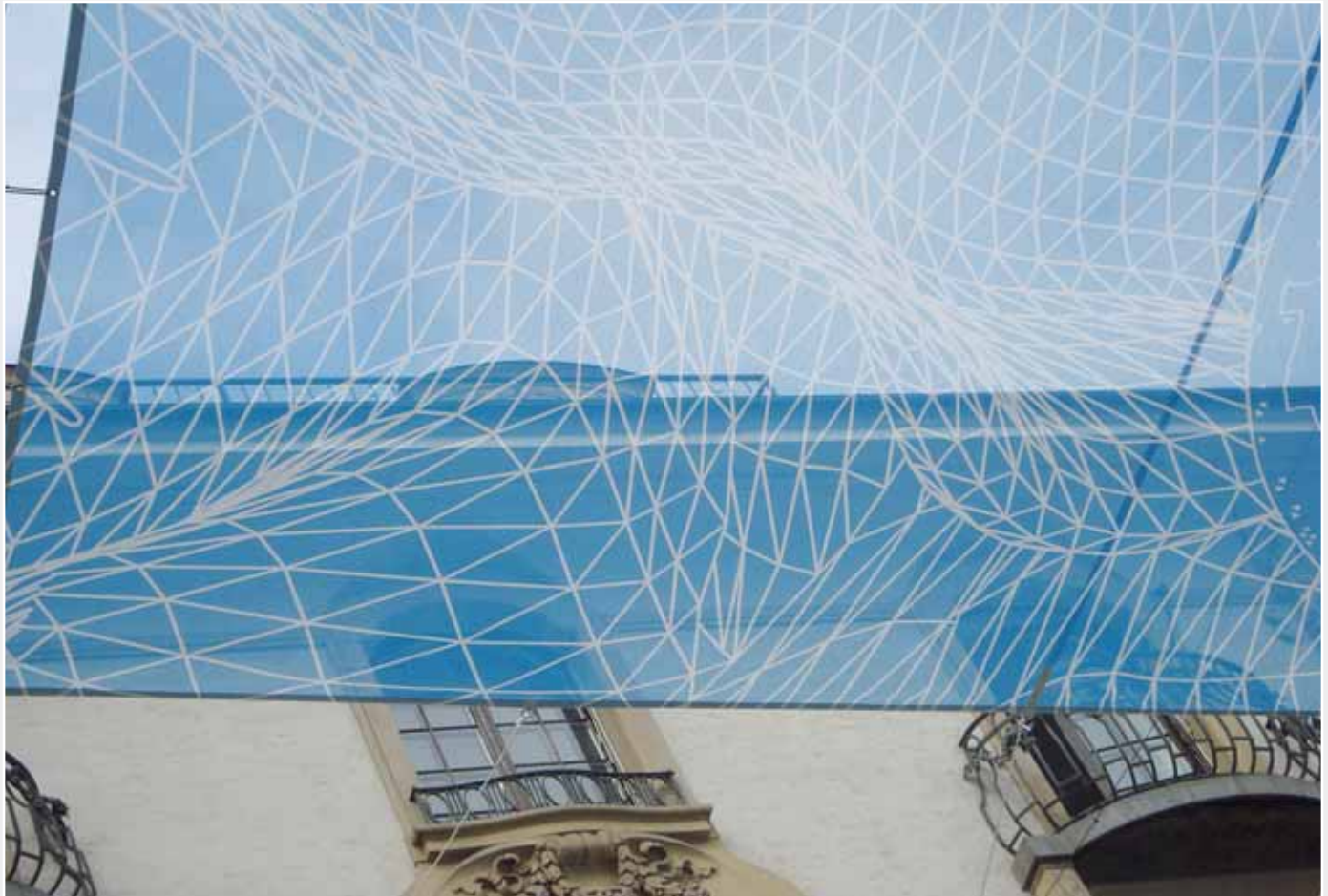
The gigantic mesh nets protect against the sun's rays and still let through enough light.
