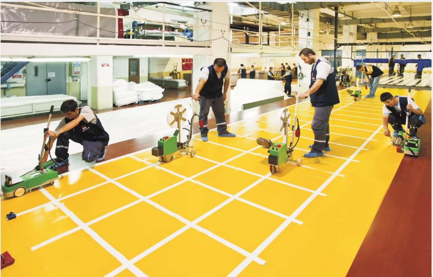
*At Kadesan, three TAPEMAT are used for the tapes and three VARIANT T1 are used for seam and overlap welding.*
