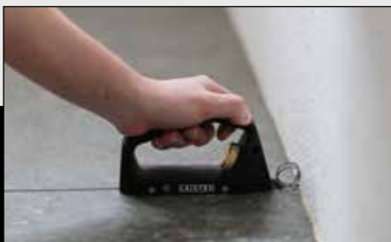
Executing clean grooves up to connecting walls
