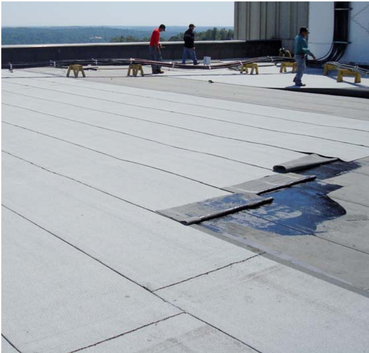
1. Open flame prohibited The safe alternative to open flame for cold applied roof systems.
