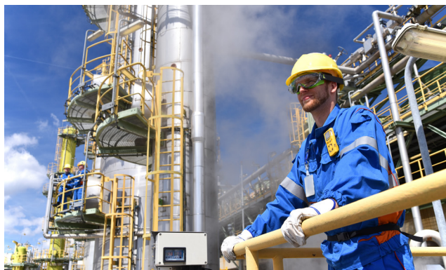
Site installation with CEM system
